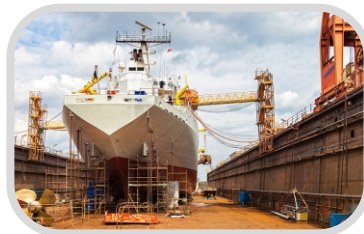
SHIP BUILDING & DRY DOCK
