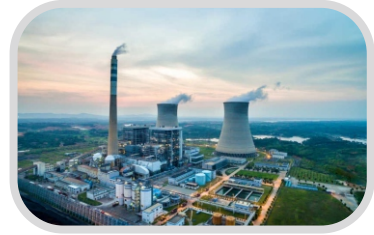
POWER PLANT SUB STATION
